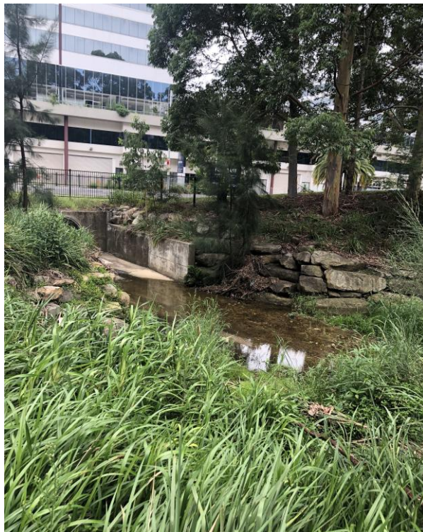
Figure 8. Area of 192 Balaclava Road (Macquarie University) land forming part of the site of the proposed works
