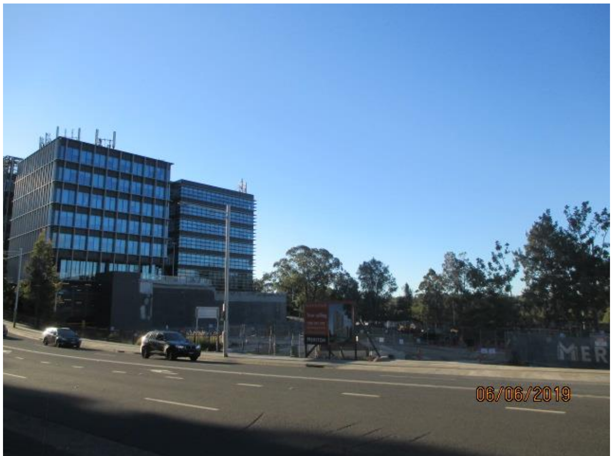
Figure 4. Photograph of the site (looking north west from Talavera Road) showing the buildings now demolished with Fujitsu building on the left
