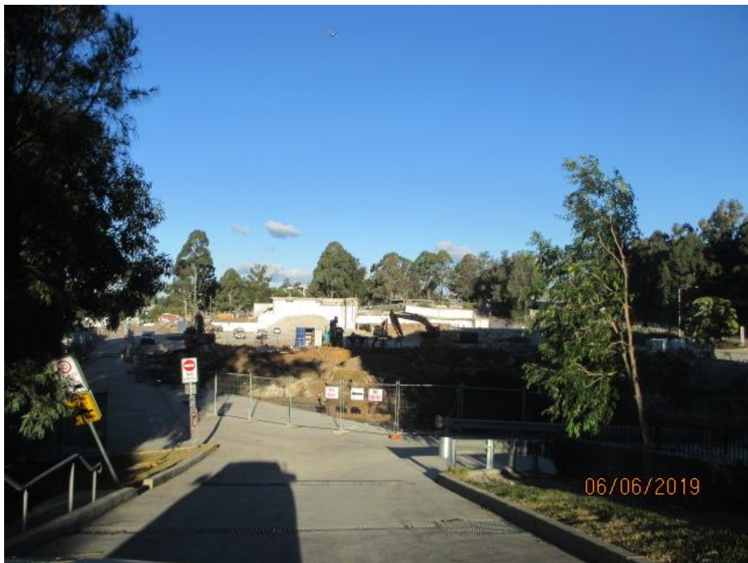
Figure 6. Photograph of the site (looking east from in front of the north of the Fujitsu building) showing the buildings now demolished. The M2 Motorway is to the left of the photograph.
